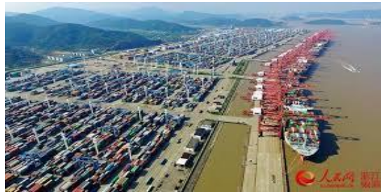
Port of Ningbo Zhoushan
